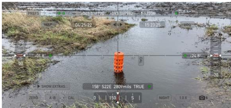
Figure 2/ Intake in the road ditch of 390th St.
