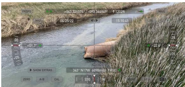
Figure 3/ Existing Tile Outlet
