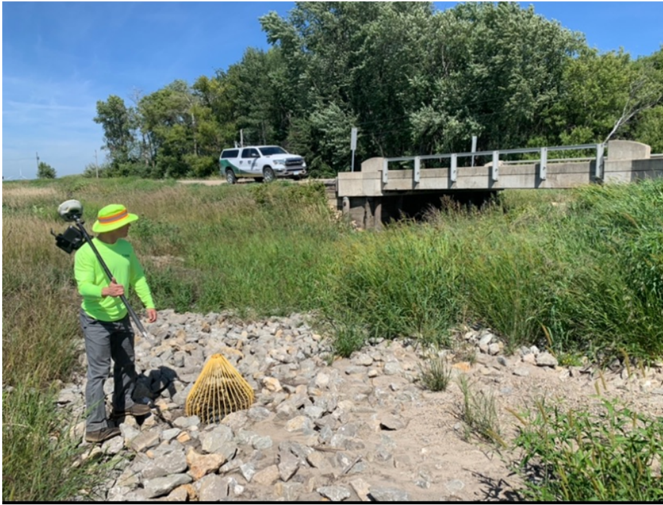
Photo 2- Intake and bridge northwest of the intersection of 105 and Vine Ave
